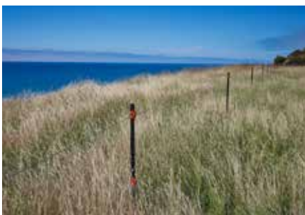
4. Put up the intermediate posts
