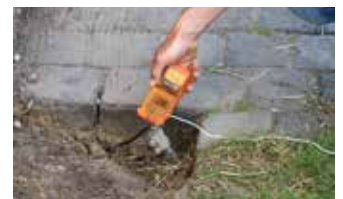
4. Check your earthing
